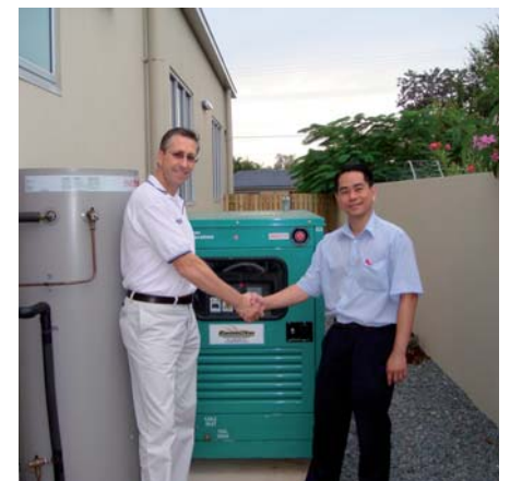
Steve Keep (NPS QLD Sales Manager) with Dr. Kai Choong and the Generator (behind).
